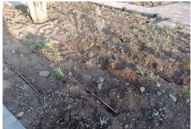
Proper in-line drip installation — before growth.
